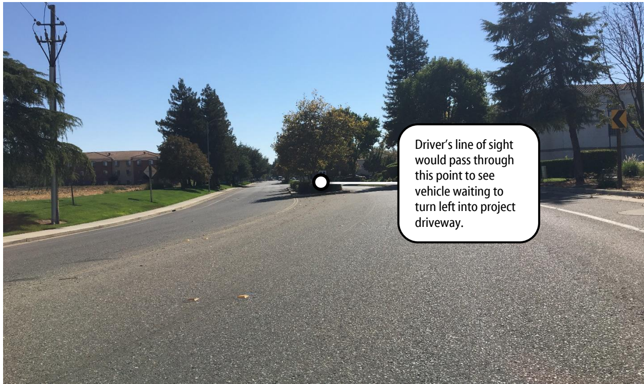
Image 3. View of median landscaping obstructing stopping sight distance between southbound motorists on Research Park Drive and the project driveway, taken from approximate driver's eye height.
